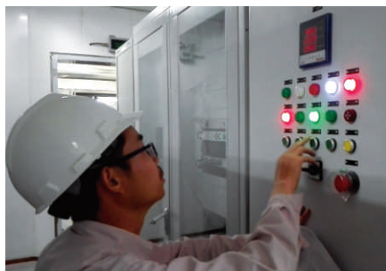
技术人员现场调试 Technical Staff On-site Commissioning
