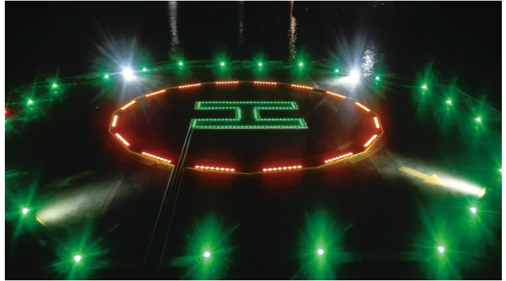
直升机平台助降系统夜景图 Night View Map of Helicopter Landing Platform Aid System
