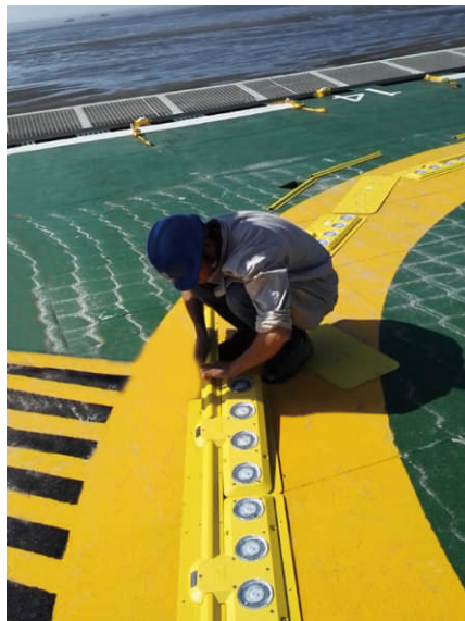
C灯现场安装 Circle Lights On-site Installation
