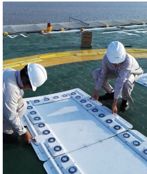
H灯现场安装 H Lights On-site Installation
